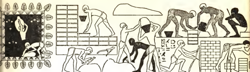
Fig. 18. Bricklaying with foreign labor in Egypt.
