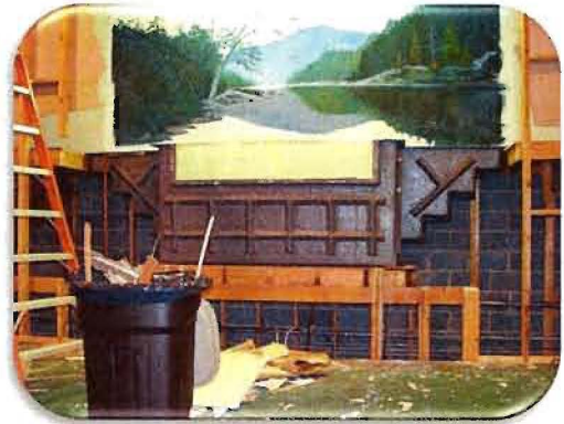
Baptistery exposed after demolition of old wall behind stage. Photo taken 2/15/10.
