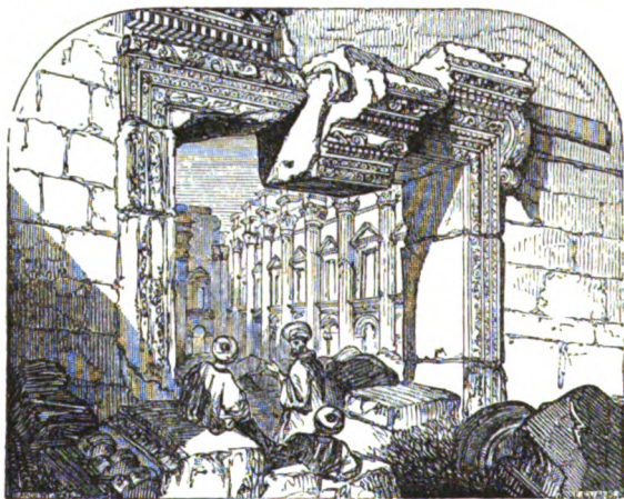
[Wall of Baalbec.—La Borde.]
